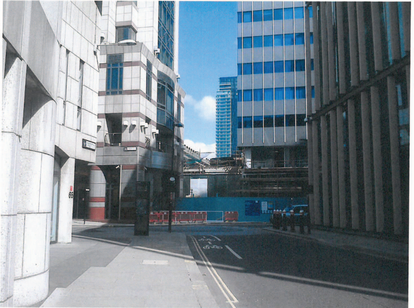
View from Basinghall Street
